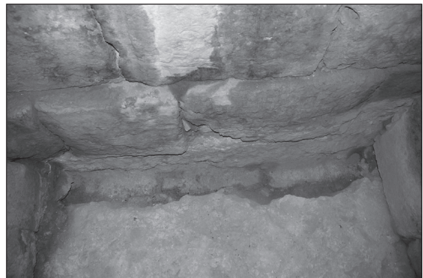
7. Southern vault under the pronaos. View of the foundation trench US18049 from top where three ashlars of the offset footing are discernible after the excavation of the fill (photo: M. Brizzi).
