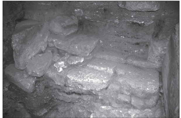
9. Central vault under the pronaos. The breach opened through foundations of the columns opening an access to the vaults from the area between the alae. In the foreground, the threshold US18058 overlaying the earlier doorstep US18024 (photo: M. Brizzi).
